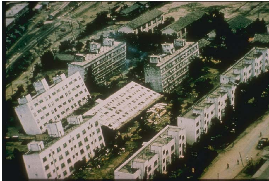
Figure 3-14: Bearing capacity failure of structures from soil liquefaction in Niigata, Japan (1964) (after NOAA/NGDC - NOAA National Geophysical Data Center).
