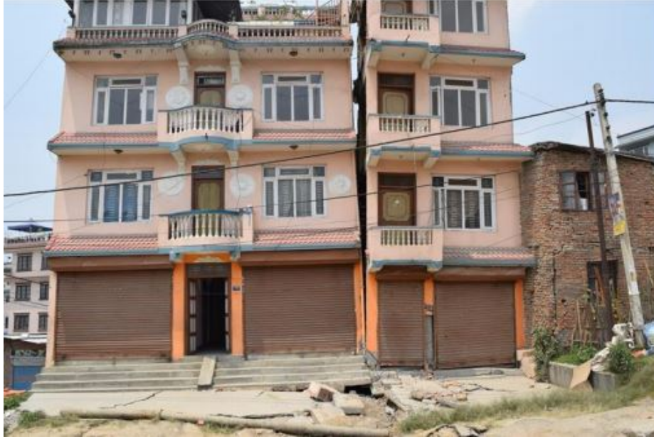
Figure 3-12: Damage to a Building due to liquefaction-induced differential settlement in Kathmandu, Nepal from 2015 earthquake event (after GEER, 2015).
