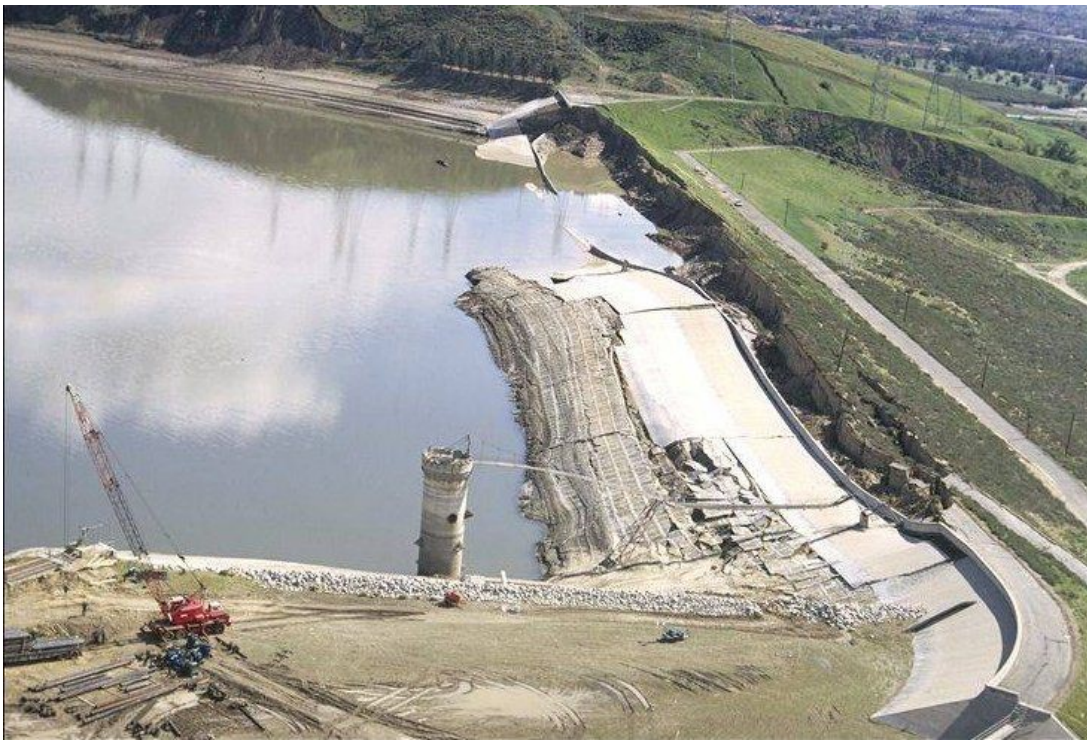
Figure 3-15: Flow liquefaction failure of the Lower San Fernando Dam, 1971 (courtesy of the National Information Service for Earthquake Engineering, EERC, University of California, Berkeley).
